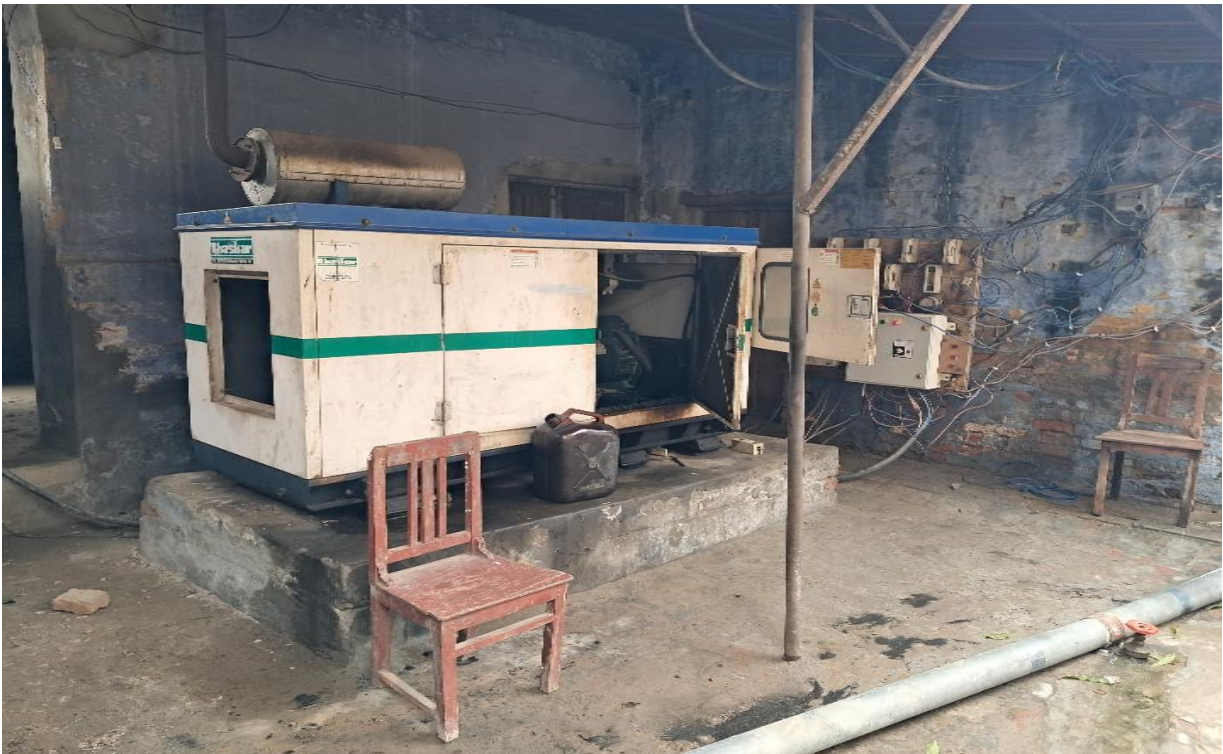
Electricity and water supply department
